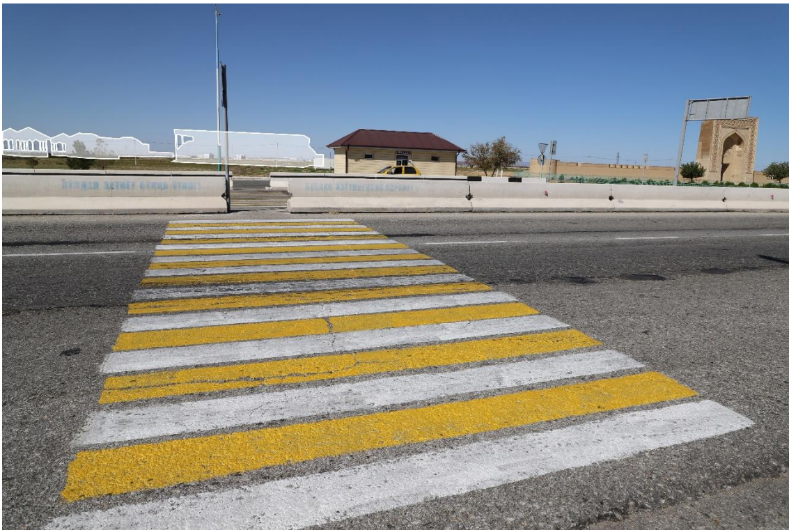
Figure 26. Visual assessment: view across the M37 motorway to the North (2). Source: IICAS, 2020
