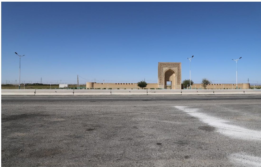
Figure 9. View to the North showing the entrance portal of the Rabati Malik Caravanserai and the location of the proposed development project. Source: IICAS, 2020
