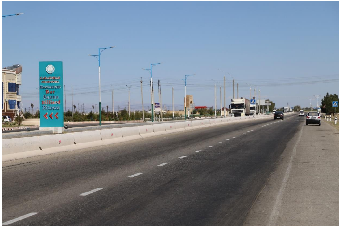
Figure 6. View to North-East toward Rabati Malik Caravanserai. Source: IICAS, 2020
