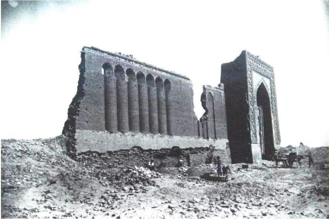
Rabati Malik Caravanserai and Sardoba: Raboti Malik Caravanserai: the repair works in 1937. Source: Ministry of Culture of the Republic of Uzbekistan (1937).
