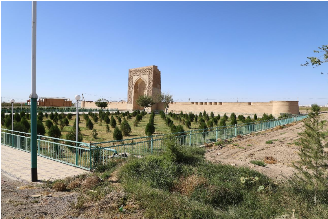
Figure 31. Visual assessment: Buffer Zone, view to the North-West (1). Source: IICAS, 2020
