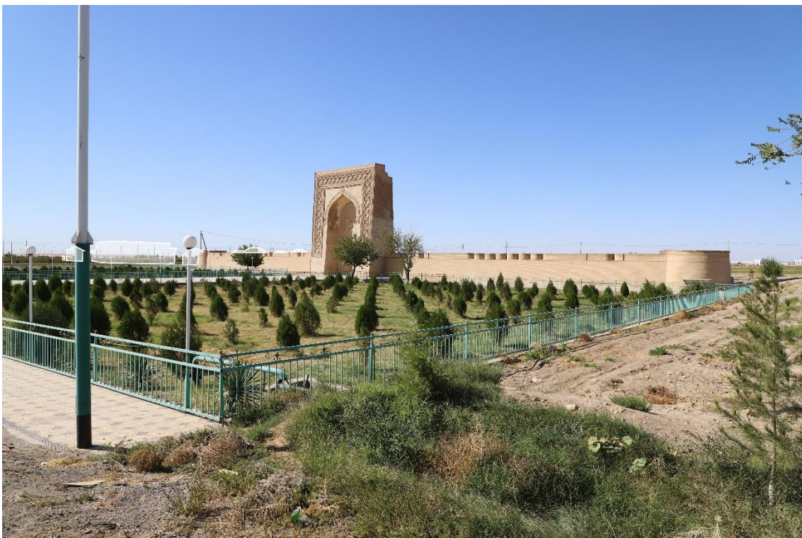
Figure 32. Visual assessment: Buffer Zone, view to the North-West (2). Source: IICAS, 2020
