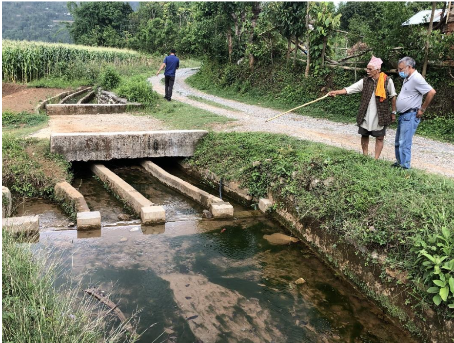
Figure 11: Current Argeli Irrigation Canal
