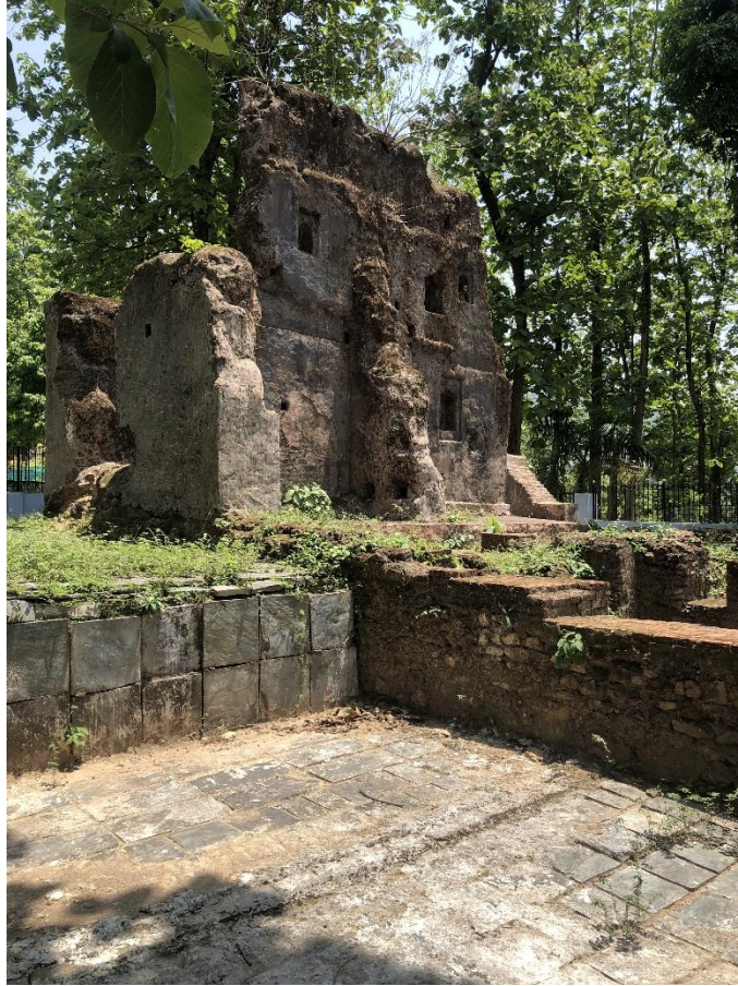
Figure 9: Front view of Sendurbar Rupture
