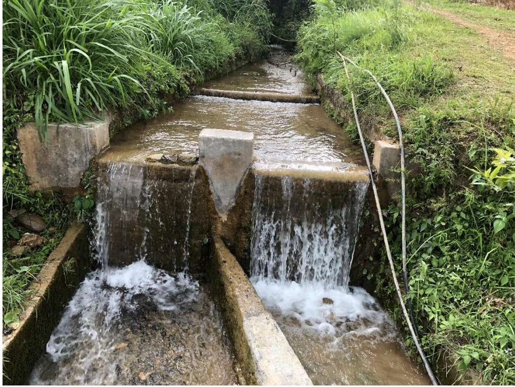
Figure 12: Current Argeli Irrigation Canal
